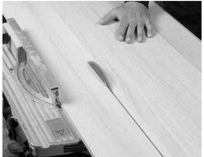
Last or first panel: saw to size.
