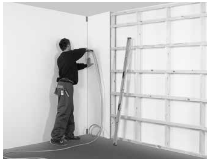
Attach it in the corner, diagonally across the panel (10 mm from the panel's edge) or with glue.
