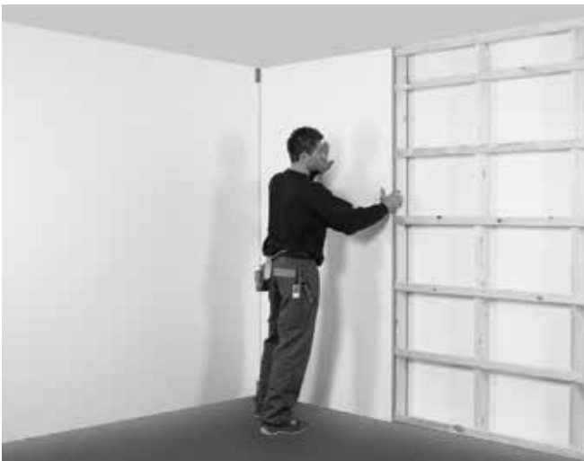
Click this panel into the previous one and attach.
