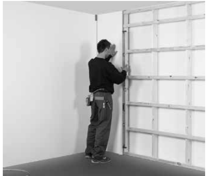
Place the first panel level.
